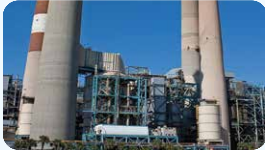
AL KHARSAAH SOLAR POWER PLANT
