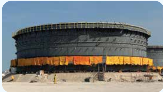
EPIC NEW GASOLINE & JET STORAGE FACILITY MIC
