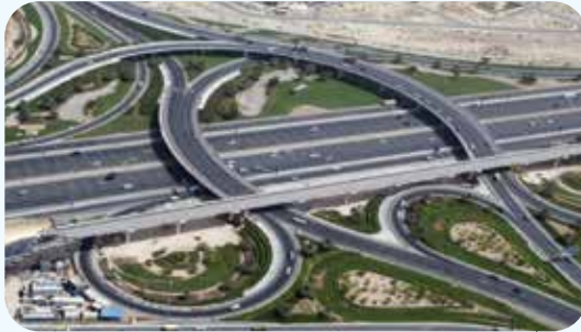
Construction of Al Rayyan Road Project 7- Contract 1
