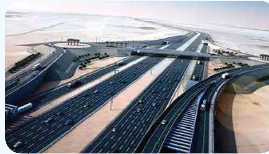
Construction of Al Khor Expressway
