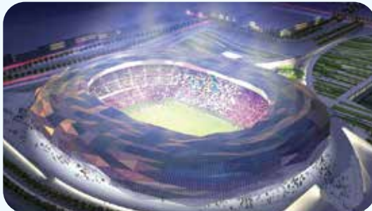
QATAR FOUNDATION-EDUCATION CITY STADIUM PROJECT
