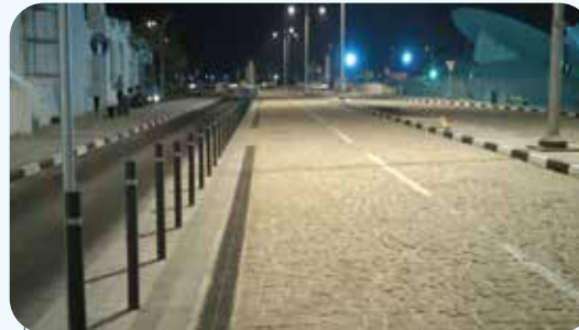
Construction of New Qatar National Museum Road
