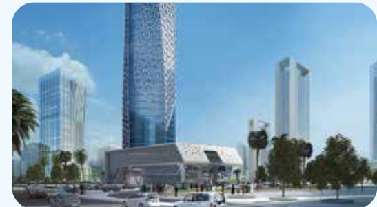
AL AHLI BANK TOWER
